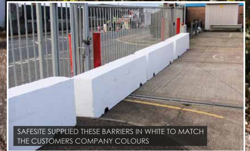
SAFESITE 3M BARRIERS PROTECTING A VULNERABLE SITE FROM FLY TIPPERS
