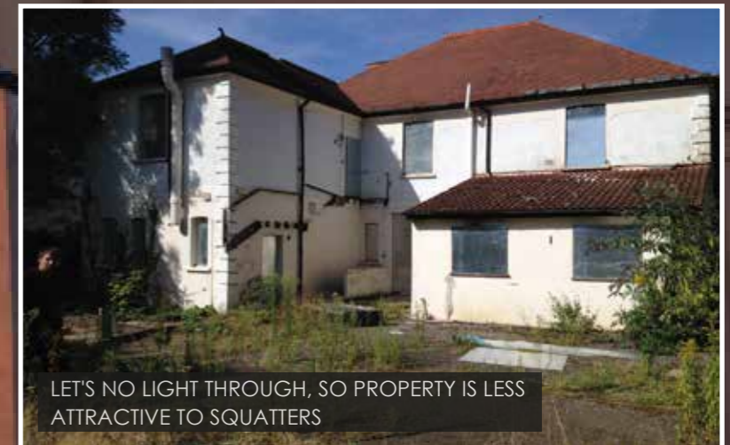
FIXED SECURELY TO THE BUILDING USING SPECIALIST SECURITY FIXINGS
